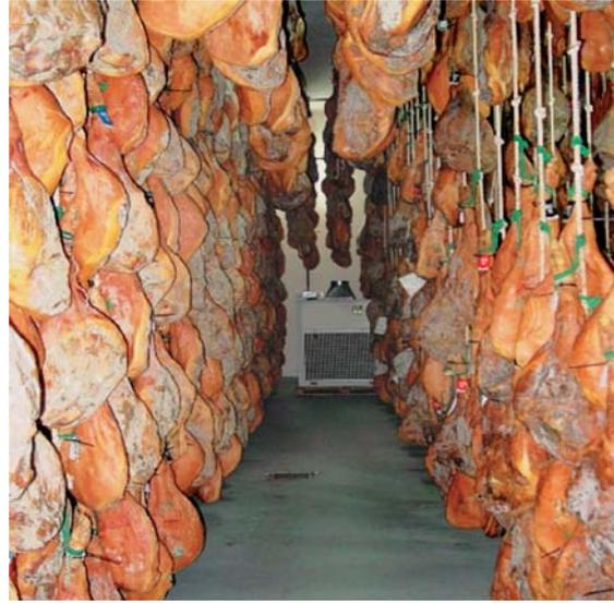
Ham seasoning plant; humidity control made by a dehumidifier model ITM400, capacity 110 l/24h, required indoor condition: temperature 15°C, relative humidity 60%.
