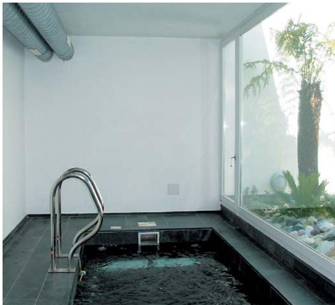
Indoor swimming pool, surface 10 m<sup>2</sup>, water temperature 28°C with health spa, humidity control made by dehumidifier model SEH160, capacity 95 l/24h. Date of installation: May 2003.
