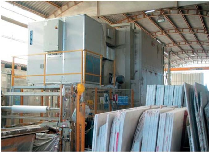
Marble resin topping plant; required process temperature 45°C, relative humidity  $\leq 15\%$ , made by dehumidifier with temperature control model KSR800. Airflow 8000 m<sup>3</sup>/h.
