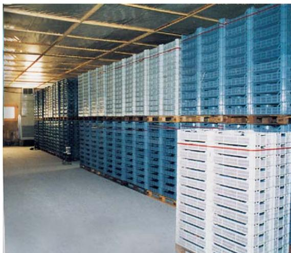
Onion preservation cold room, made by low ambient version dehumidifier model ITM400BT, capacity 60 l/24h, required indoor conditions temperature 2°C, relative humidity 60%. Date of installation: May 2003.
