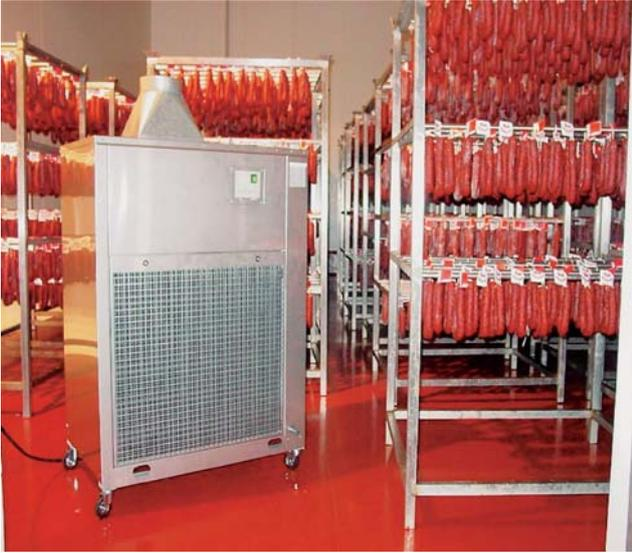
Salami seasoning plant; humidity control made by a dehumidifier model ITM330S in stainless steel, capacity 90 l/24h, required indoor conditions: temperature 15°C, humidity 60%.
