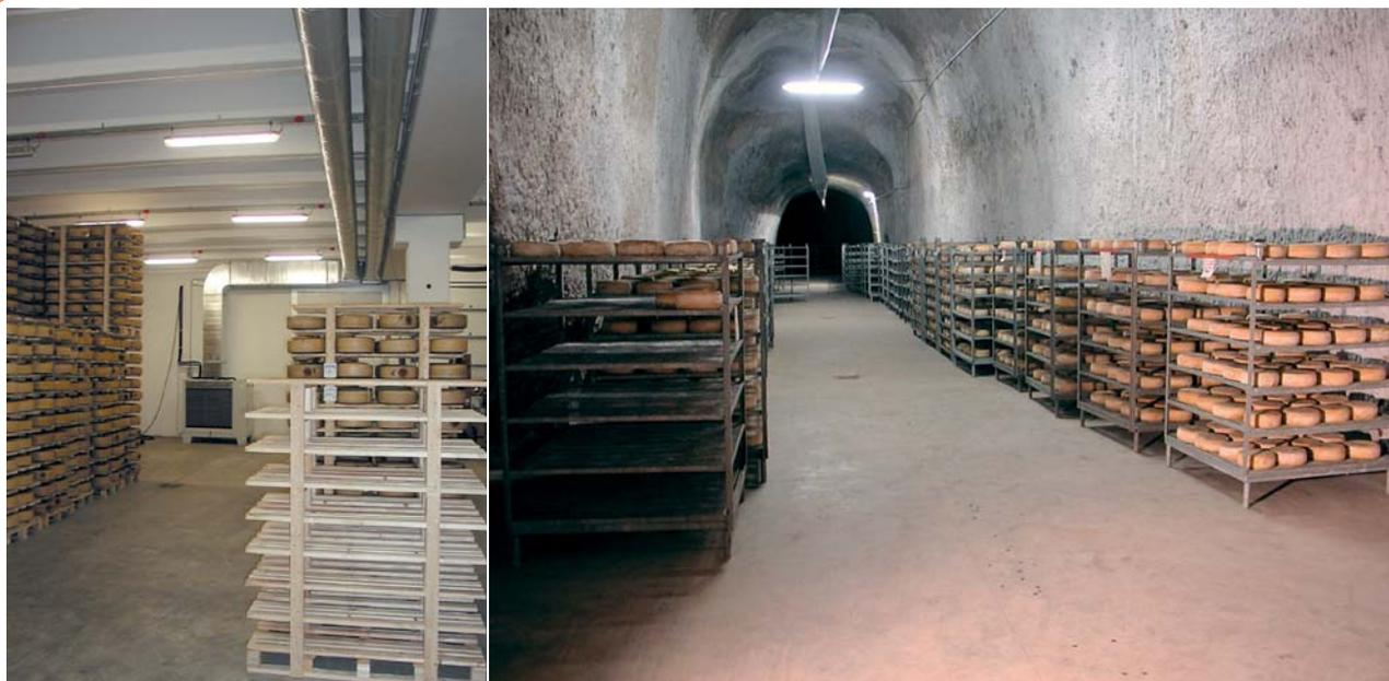
Cheese seasoning storage plant, made by dehumidifier with temperature control and remote condenser model FLZ740. Required room temperature 18°C, relative humidity 70%. Date of installation: May 2003.
