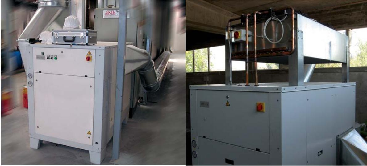
Industrial water base painting process; drying process made by dehumidifier model FL940, required temperature 30°C, airflow 8000 m<sup>3</sup>/h. Date of installation: January 2005.
