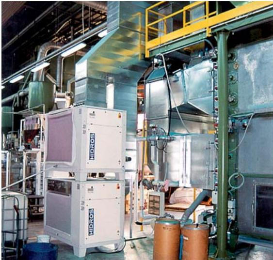
Industrial drying plant; required relative humidity  $\leq 55\%$ , made by two dehumidifiers model FL940, total airflow 16400 m<sup>3</sup>/h.
