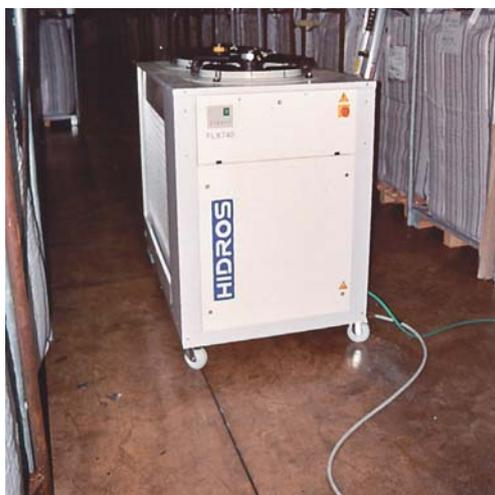
Hazelnut preservation cold room, made by eight low ambient version dehumidifiers model FL940BT, capacity 720 l/24h, required indoor conditions: temperature 2°C, humidity 60%. Date of installation: July 2004.
